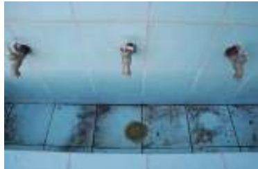
Fig 11. New taps installed, with plastic mesh protecting the plug hole from blockage by debris.
