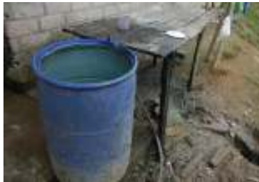
Fig 7. Drum and outlet pipe from pump behind comedor. The table is used for washing up. Some grey water puddles in the uneven surface below the table.
