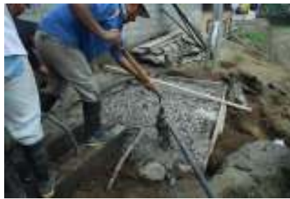
Fig 23. Minga. The base is filled in and concreted.
