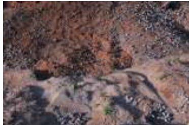
Fig 14. Finished soakaway back filled with excavated earth.
