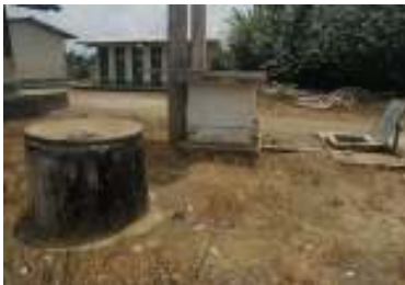
Fig 4. Headstone with cover. Visible beyond the well are the cistern and housing for the pump that was used to pump water from the cistern to the water tower.
