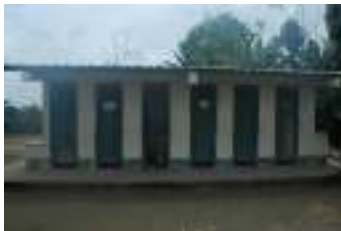
Fig 1: Block of latrines
