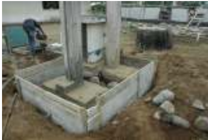
Fig 17. The trench is dug ready for concrete to reinforce the base
