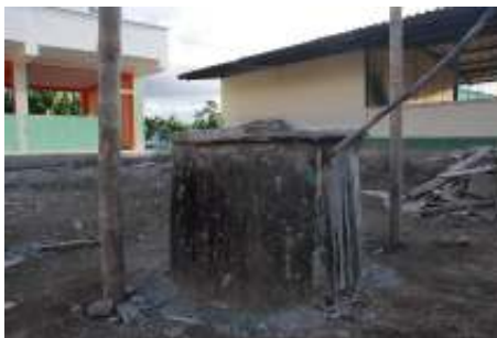
Fig 16. Well with the outlet pipe exiting via a hole in the side of the headstone.
