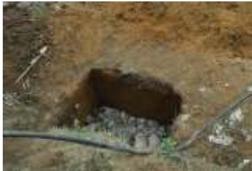
Fig 13. Soakaway pit under construction
