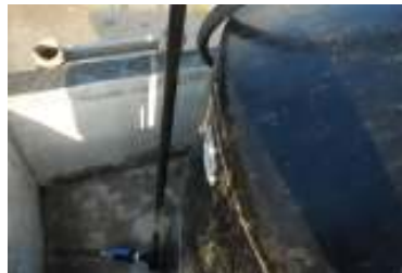
Fig 19. Ladder in position providing access to the tank for water treatment.
