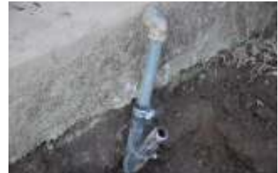
Fig 12. Simple method of blocking the second inlet to the toilet back plumbing to 'close the loop' and stop leakage/pressure loss.
