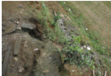
Fig 8. Grey water draining down from the washing station and accumulating on the ground below.
