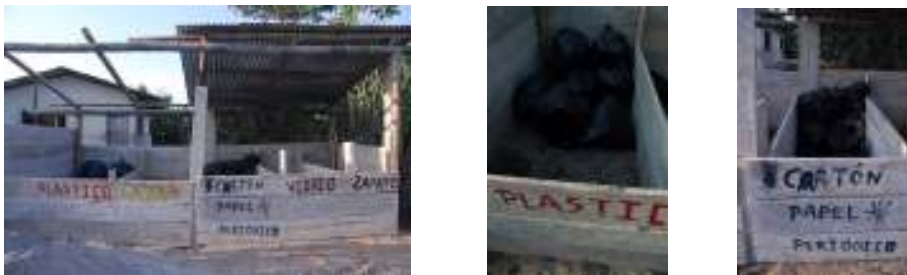
Fig 3 - 5. Centro de acopio as at Thur 6 th Sep. Further work is required to complete the roof on the left hand side of the structure. This could either be done through the purchase of more tin roofing sheets, or alternatively using a more traditional roof built from woven palm leaves as in fig 6.
